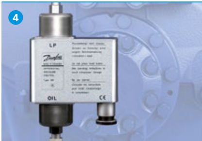
Oil pressure safety switch
